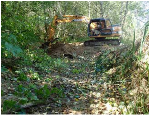
Barrier culvert removal project, Morris Creek. Photo: Seth Mead.
