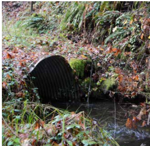
Culvert to be replaced on Deadwood Creek.
