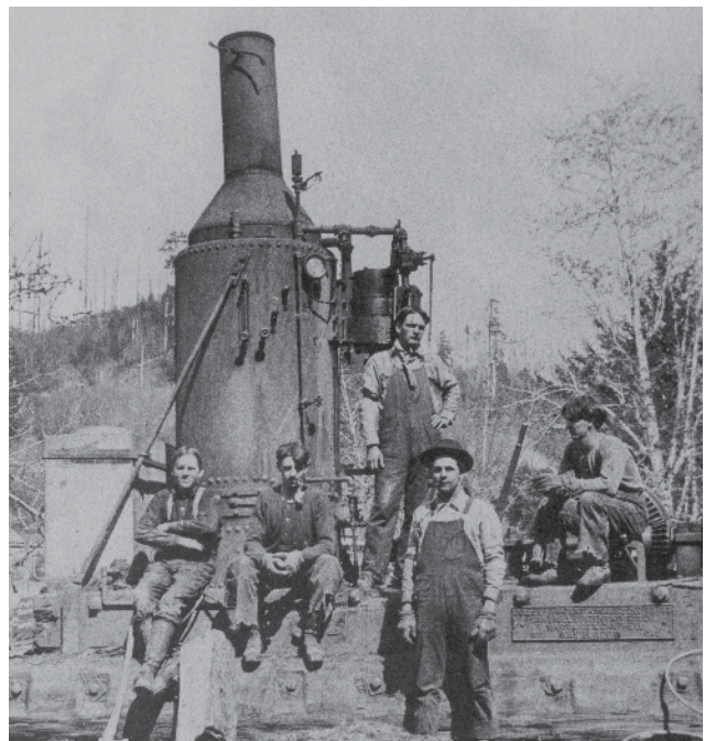
In use from the 1880-1930s, steam donkeys greatly improved the efficiency of logging in coastal watersheds. Photo: Florence Pioneer Museum.
