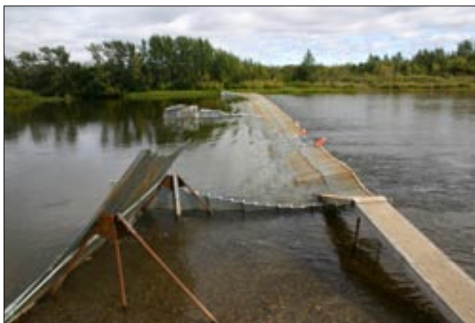
FIGURE 2. — A resistance board weir featuring a skiff gate to allow boat passage (in the foreground, marked by pylons), a trap to capture fish in middle of weir, and a passage chute (background), where fish are counted as they pass the weir. Pilgrim River, Alaska. (Photo: Karen Dunmall and Tim Kroeker.)
