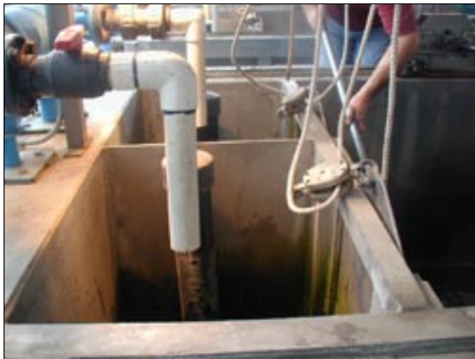
FIGURE 6. — Sample tank pre-anesthetic chambers at the McNary Juvenile Fish Facility.
