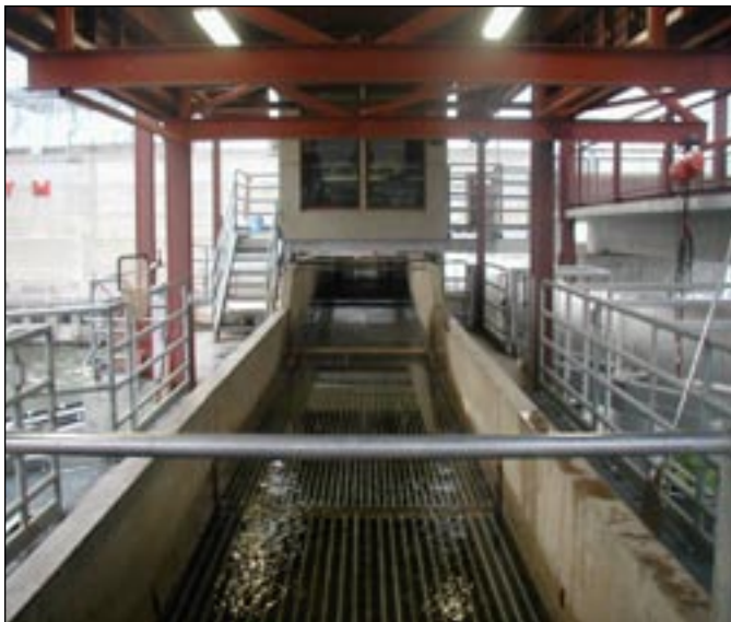
FIGURE 4. — Juvenile fish facility bar separator at the McNary Juvenile Fish Facility.
