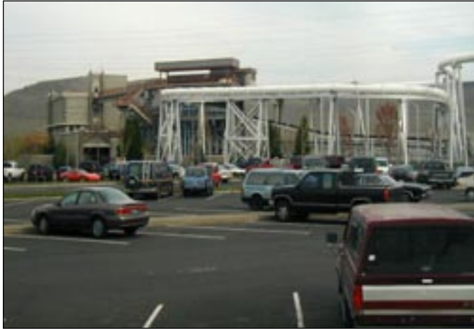
FIGURE 3. — McNary Dam juvenile fish collection facility.
