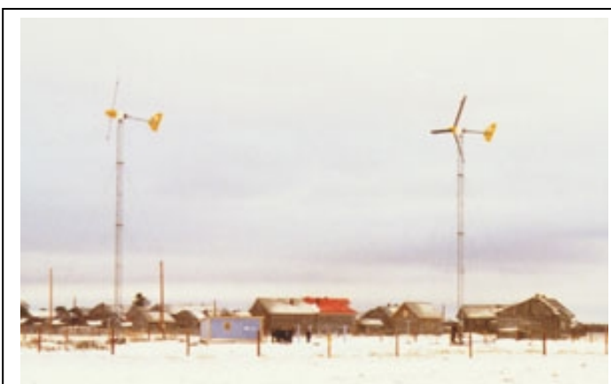
A model for Kamchatka? 7.5 kW wind-diesel hybrid turbines for community electrification, Krasnoe Island, Archangelsky District (Bergey Windpower Co.)
