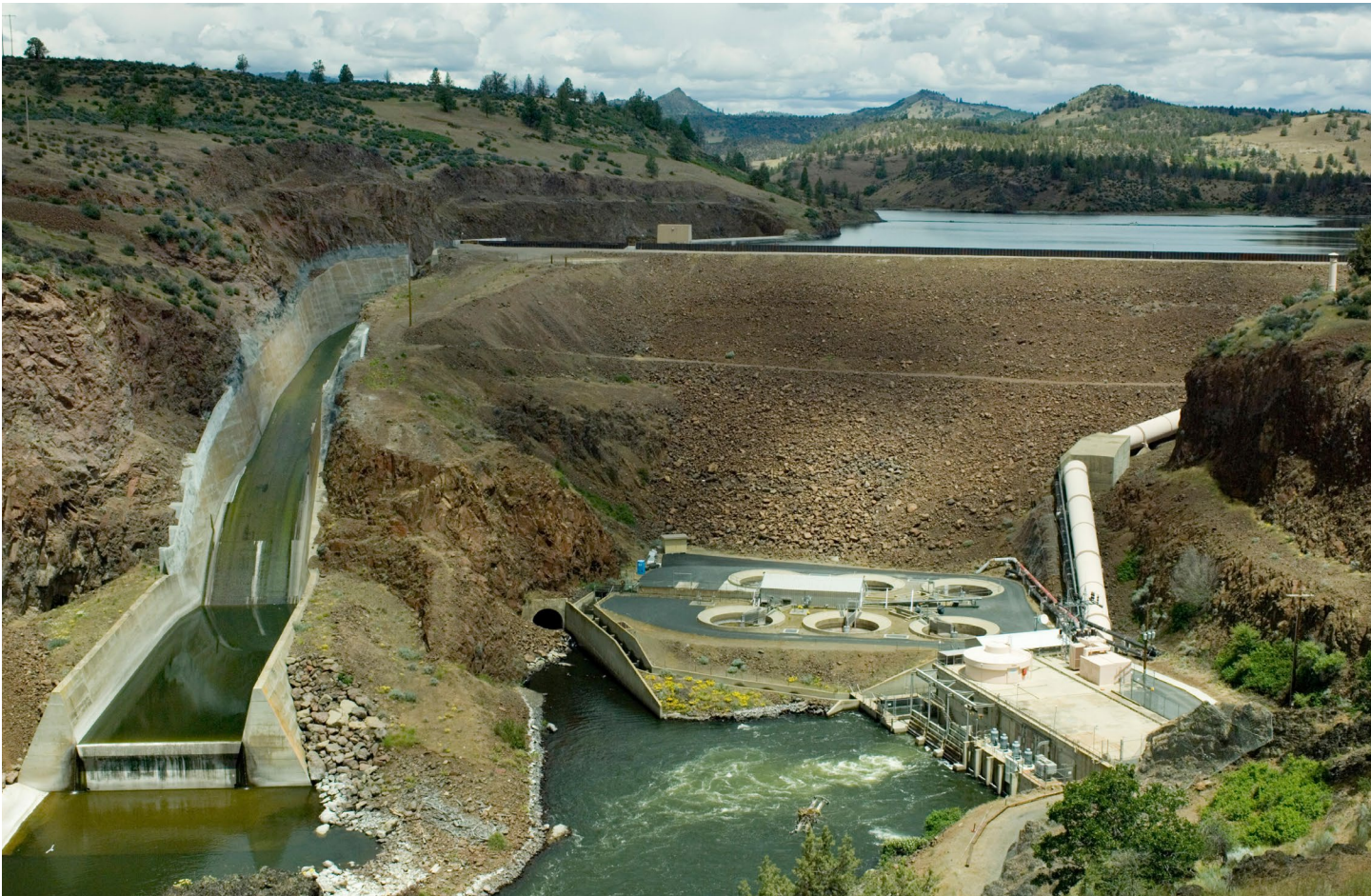
The Iron Gate Dam soars 170 feet above the Klamath River. Built without fish passage, it blocks migrating salmon. (PC: Alamy)
