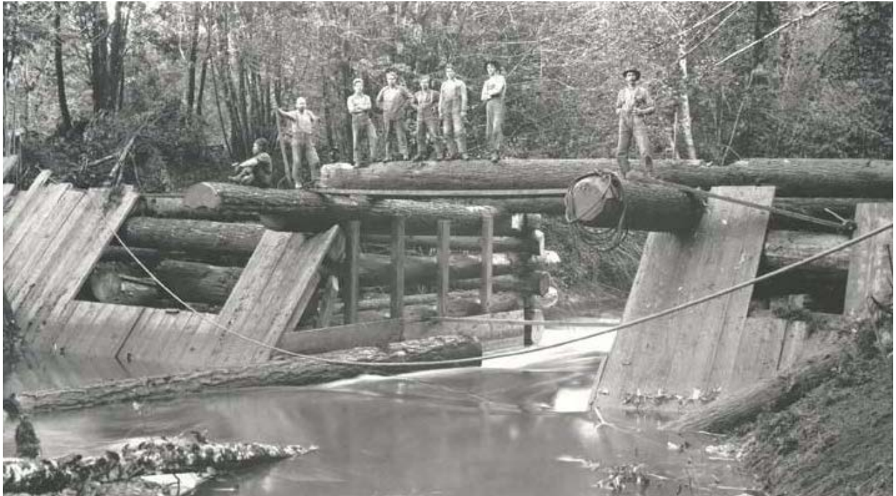
Figure 5.1.1. North Fork Coquille River splash dam. Photo: Emily Ronnow.
