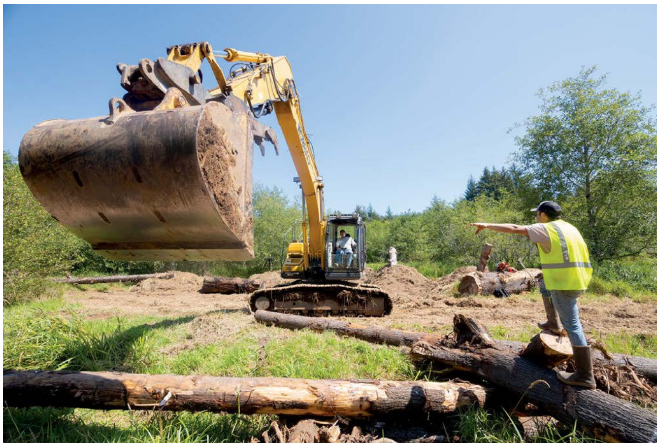
Restoration practitioners placing large wood at a tidal estuary project. Photo: Josh Havelind
