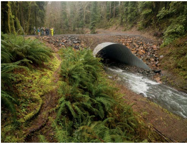
Newly installed 50 ft culvert on North Creek in the Siletz watershed. Photo: MidCoast Watersheds Council
