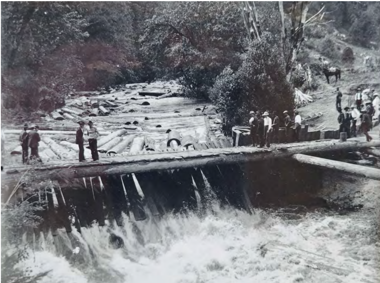
Another splash dam on the North Fork Coquille River used to transport logs downstream to sawmills. Photo: Emily Ronnow.
