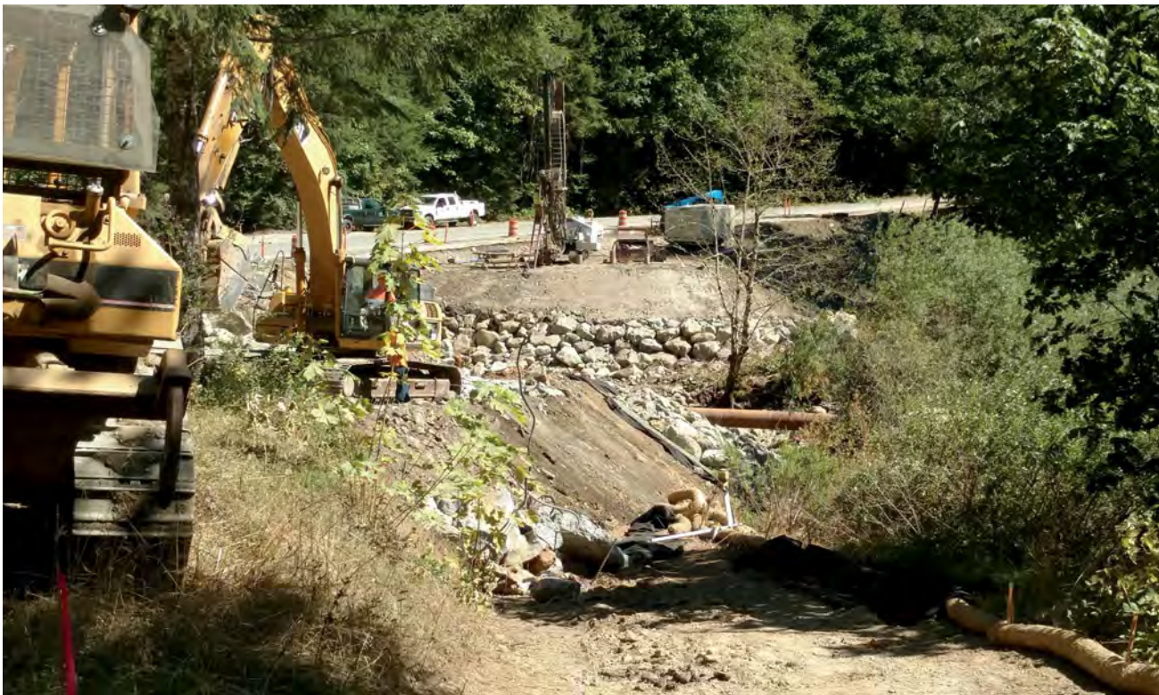
Restoration project on Coal Creek. Photo: ODFW.
