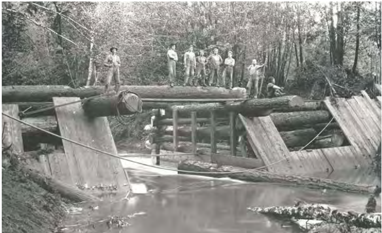
A splash dam on the North Fork Coquille River was used to raise the water level and float logs downstream to sawmills. Photo: Emily Ronnow.
